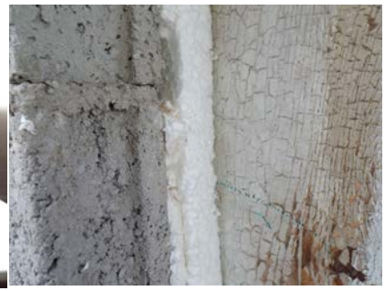
heat-insulated walls with foam polystyrene tiles
